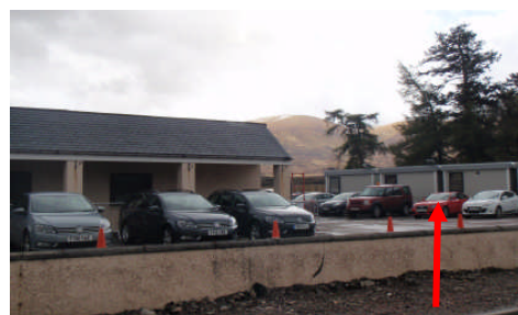
Fig. 4 : Portacabins in place
